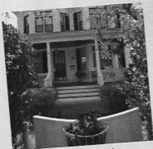
Number 26 Greenough Place, a three-story, five-bedroom Colonial Revival, was built in 1903.
